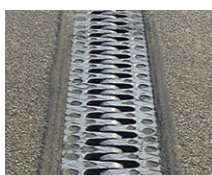
Cantilever finger joint
