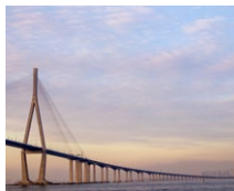
Incheon Bridge (KR)
