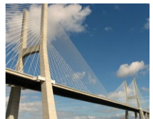
Vasco da Gama Bridge (PT)
